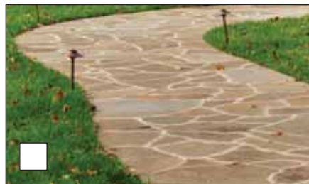
WET LAID FLAGSTONE
