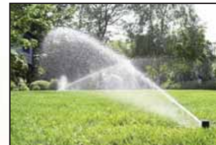
Automatic irrigation system.
