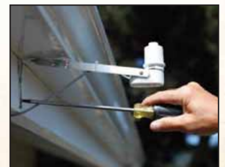
Automatic irrigation rain sensor.
